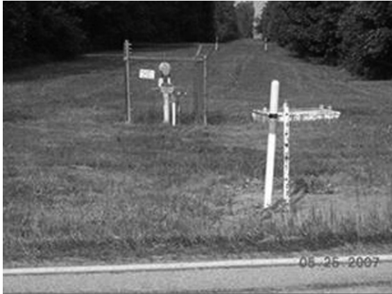
8.8 Pipeline right-of-way in good condition for CIS.
