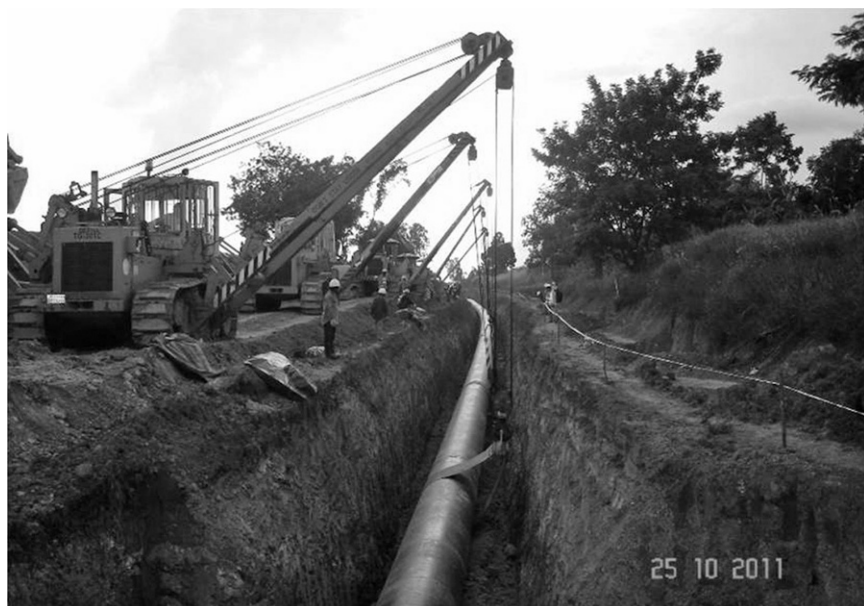
3.1 Transmission pipeline being constructed.
