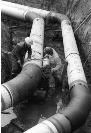
3.3 Pipelines are surrounded by earth that can lead to external corrosion.
